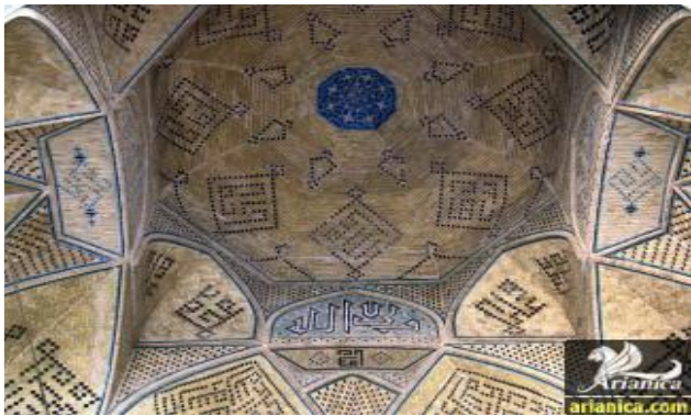
Figure13: Roof cover of the east porch of Abbasi Mosque (Source: Author)
