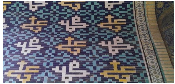
Figure 20: north prach. (Source: Author).
