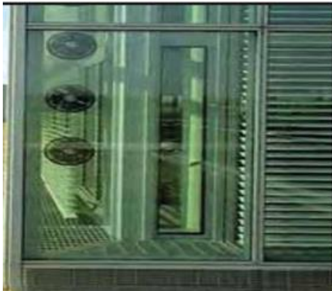
Figure (4) the Double Façade [21]
