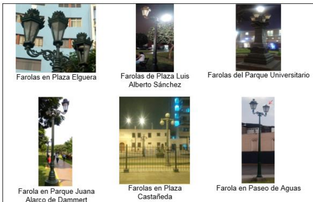
Figure 2. Main failures in lighting systems in squares and parks in the Historic Center of Lima, 2019.
